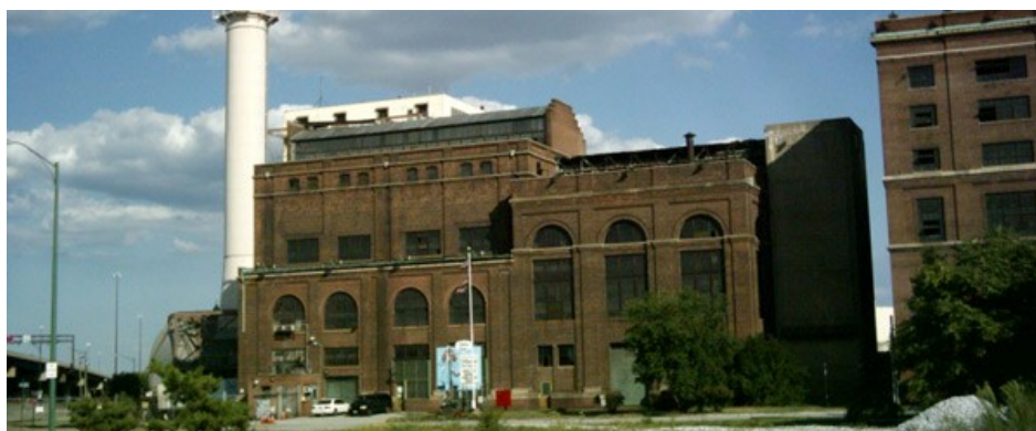
Constellation's Gould Street generator is one of the resources providing reactive power in PJM's BGE zone.
