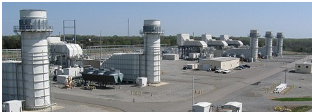
Ladysmith Power Station | Dominion
